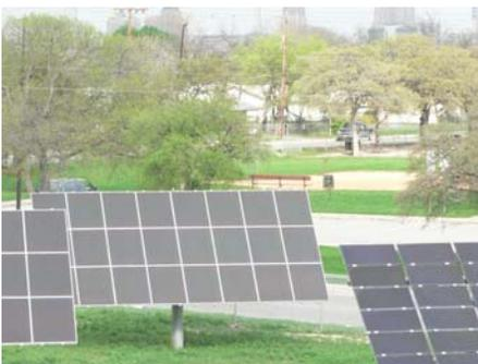
The photovoltaic system features amorphous silicon thin film modules and Copper Indium Gallium Di-Selenide (CIGS) thin film modules, supported on Roof Top (RT), Top-of-Pole (TP), Vertical Single Axis Tracker (VSAT), and Dual Axis Tracker (DAT) structures. The peak power generation capacity of the system is 48.8 kW<sub>DC</sub> or 42.5 kW<sub>AC</sub>. The estimated annual energy production is 80,000 kWh<sub>AC</sub>.
